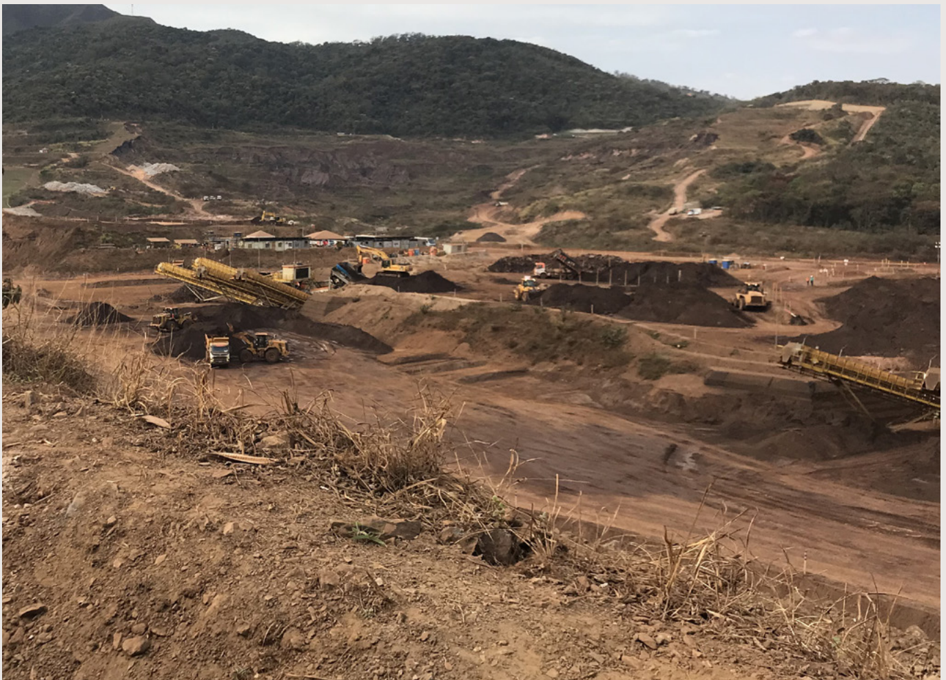
The collapsed tailings dam at Brumadino and the excavations taking place to find the four remaining bodies
